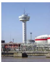
游山雷达站 Youshan Radar Station
